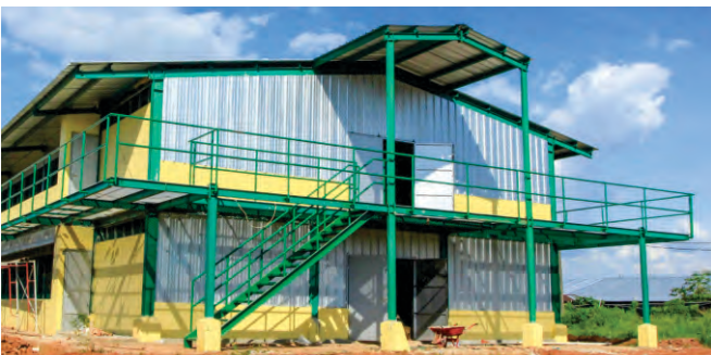
Project Name : FARMER BUILDING Client Name : PT. Charoen Phokpand Tonnage : 150 MT Location | Year : Bogor, West Java - Indonesia | 2014
