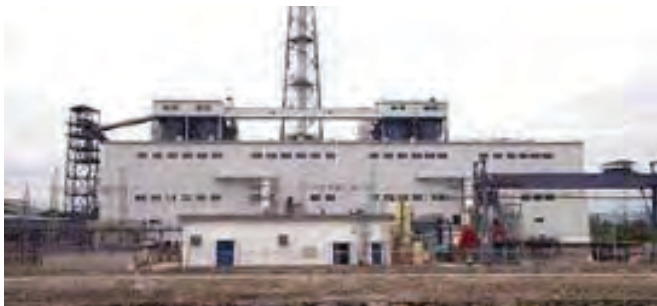
Project Name : PLTU 150 MW - Coal Fired TeiSei Client Name : Daiho Corporation Tonnage : 520 MT Location | Year : Mindano - Philipine | 2010
