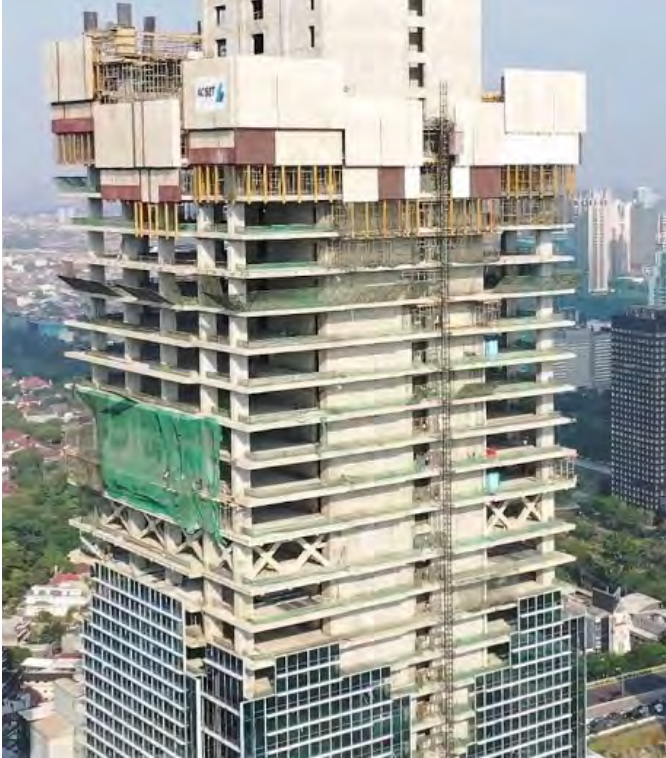
Project Name : THAMRIN NINE (Belt Truss & Outrigger) Client Name : PT. Putragaya Wahana Tonnage : 2550 MT Location | Year : DKI Jakarta - Indonesia | 2018
