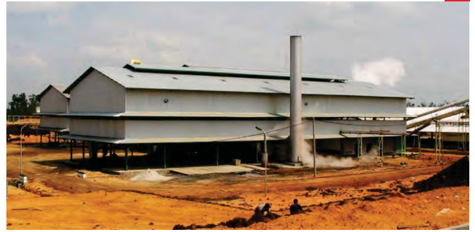
Project Name : CRUDE PALM OIL (CPO) BONTANG MILL Client Name : PT. Polasihan Prima Lestari Tonnage : 430 MT Location | Year : Palembang, South Sumatera - Indonesia | 2000
