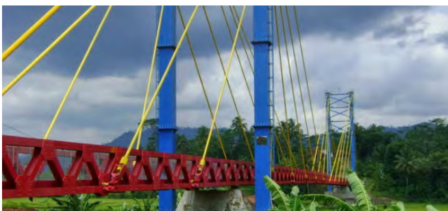
Project Name : PROTOTYPE JEMBATAN CABLE STAYED Client Name : PT Waskita Karya Wilayah Tengah Tonnage : 206 MT Location | Year : Sukabumi, West Java - Indonesia | 2009
