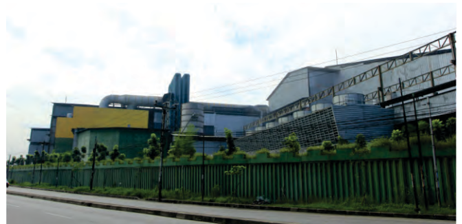
Project Name : FACTORY & WAREHOUSE GG3 Client Name : PT. Gunung Garuda Tonnage : 600 MT Location | Year : Bekasi, West Java - Indonesia | 2013
