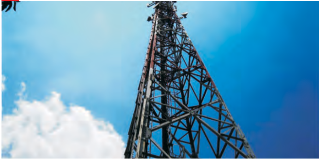
Project Name : TOWER INDOSAT Client Name : PT. Bahayutama Kerta Mukti Tonnage : 94 MT Location | Year : Jakarta - Indonesia | 2002
